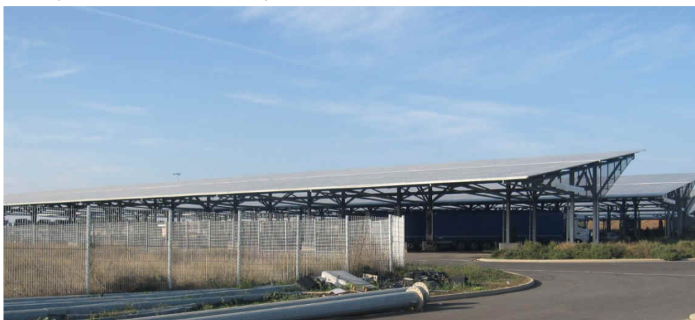
Figure 163 : Ombrières photovoltaïques (Via Europa) (Source : AMAE)
